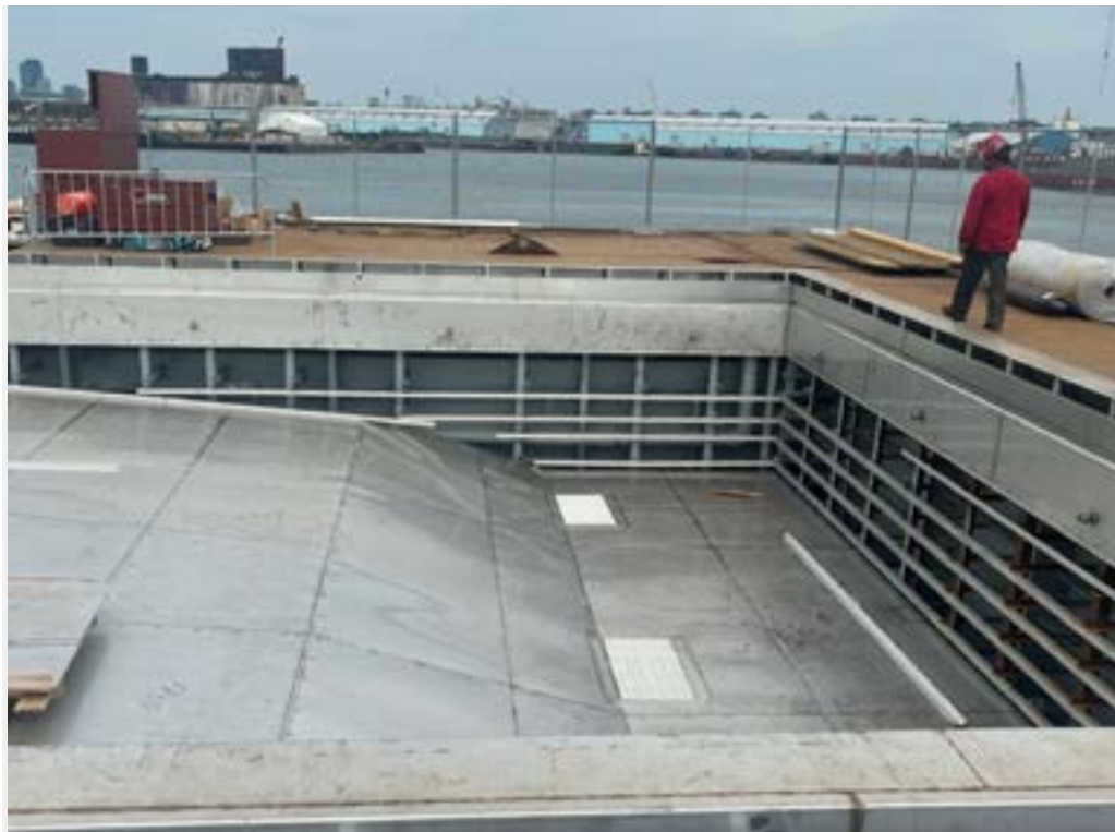
POOL1 pilot pool under construction at the Erie Basin Bargeport in Red Hook, Brooklyn. Photo courtesy Friends of + POOL, 2026.
