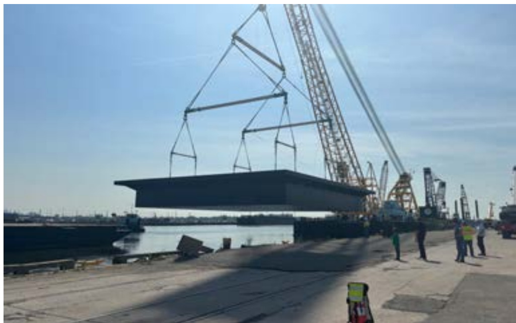
The 320 ton shell of the pilot + POOL was craned into the water at Port Newark, July 30, 2025. Courtesy Friends of + POOL.
